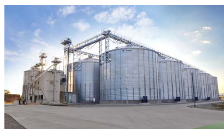
Grain drying facility
